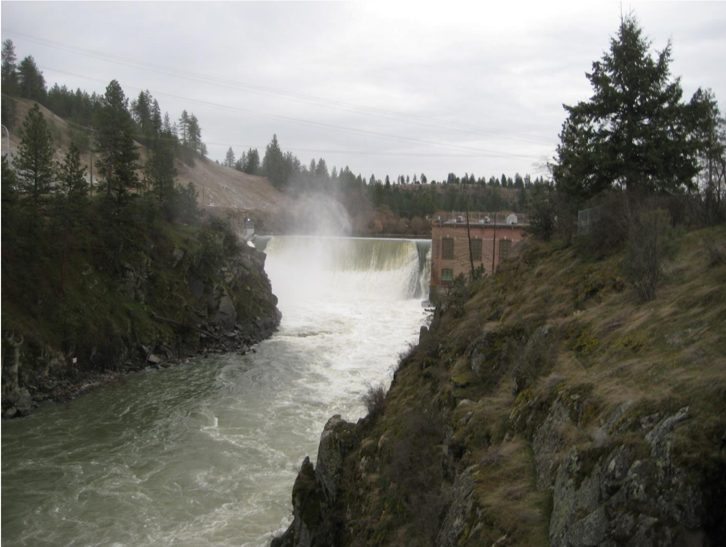
Figure 2-1: Photograph of Nine Mile Dam with Pneumatically Controlled Metal Gate, March 24, 2011 (approximate discharge 11,400 cfs from spillway and 13,800 cfs total)
