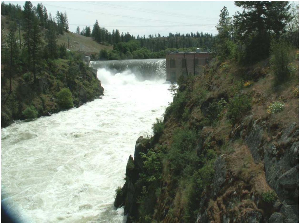
Plate NM1. Nine Mile Dam and Powerhouse Viewed From West Charles Road Bridge, May 22, 2008 at 11:15 PDT
