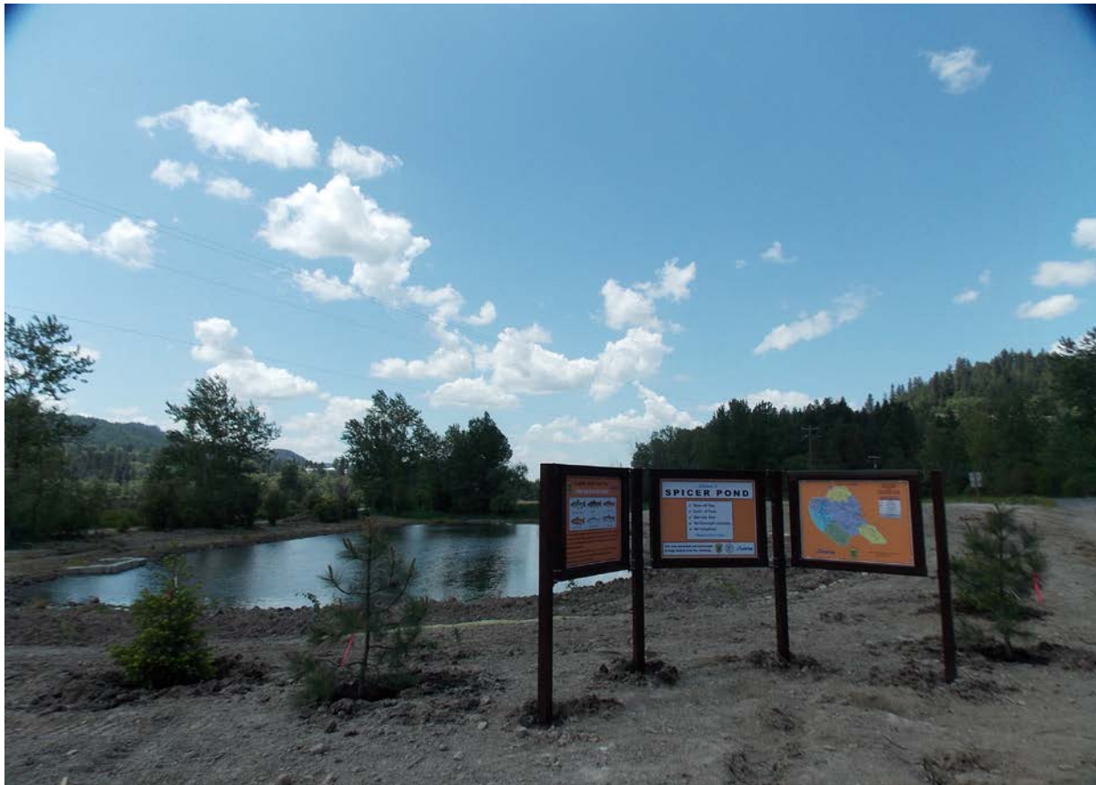
Figure 7. Spicer Pond Construction and Information Kiosk, Summer 2014
