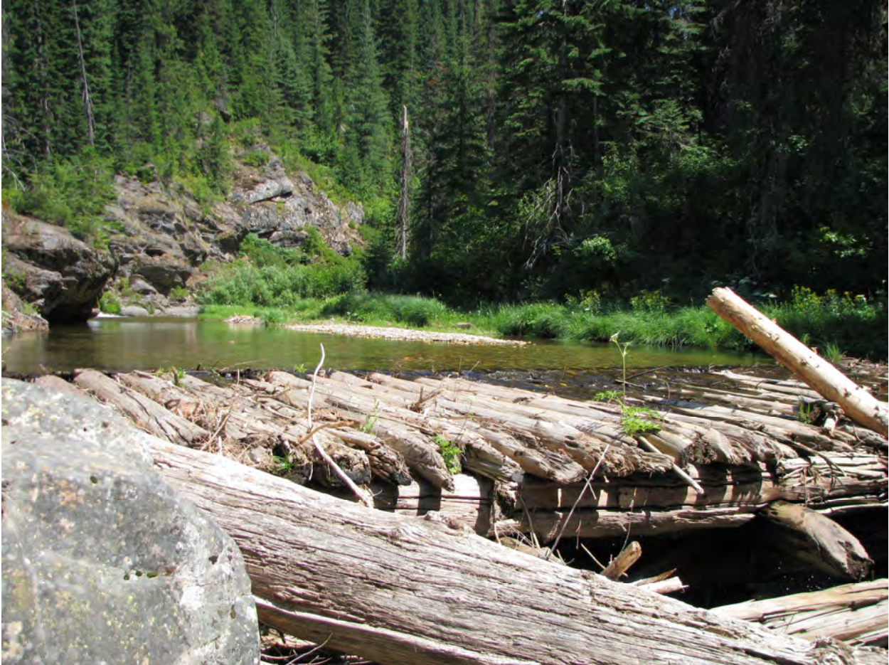
A top view of Splash Dam 3, looking upstream in Marble Creek, Idaho, on July 27 2007.
