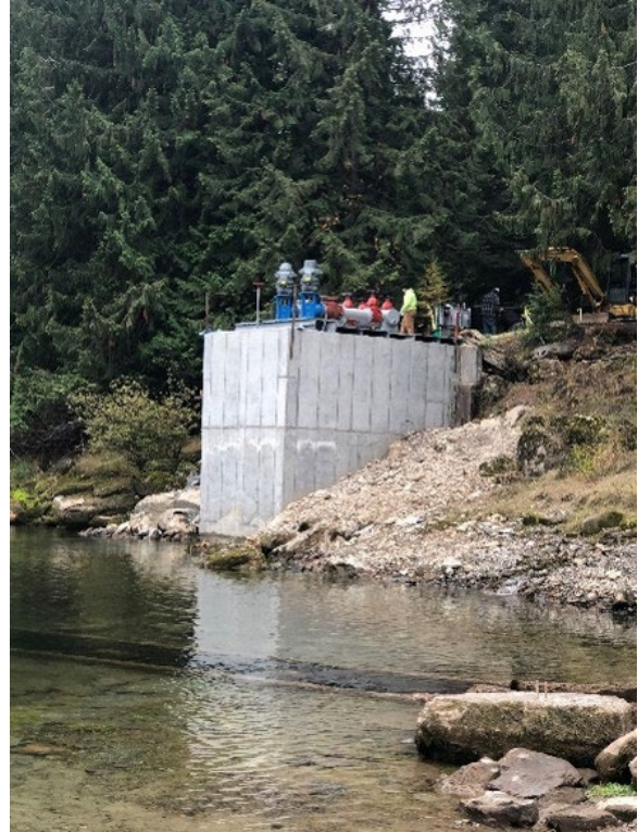
After construction photo of the new collection basin and equipment.
