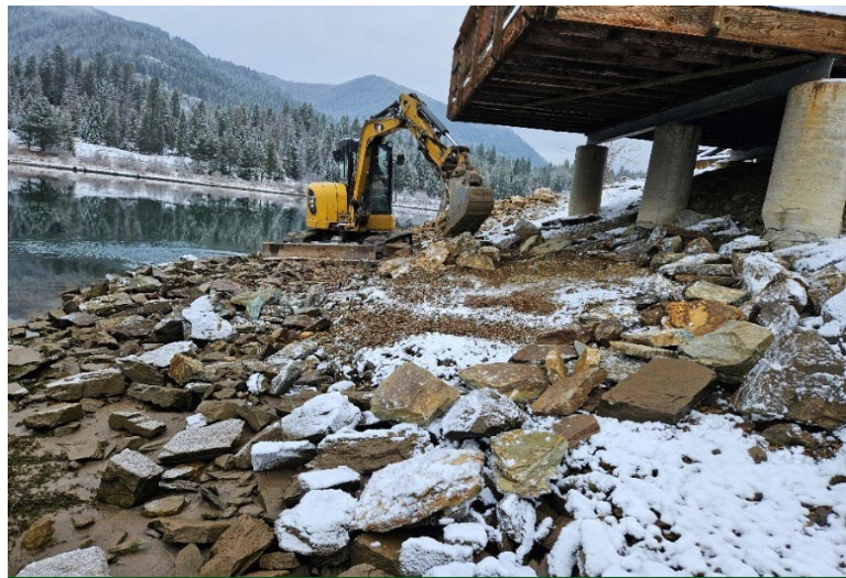
Shoreline stabilization construction under the Pilgrim Creek Park fishing platform.
