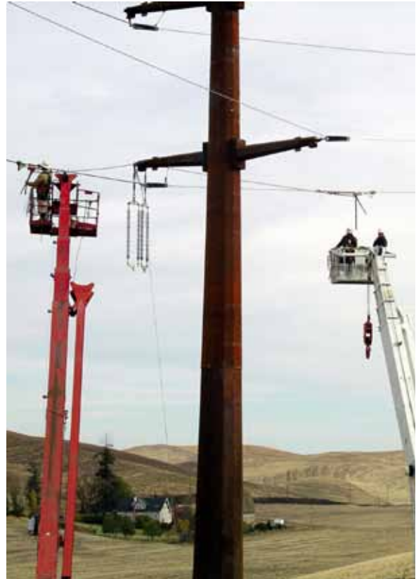
Transmission upgrade work
