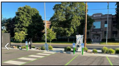
180kW DCFC at The HIVE in Spokane, WA – expandable to 1MW
